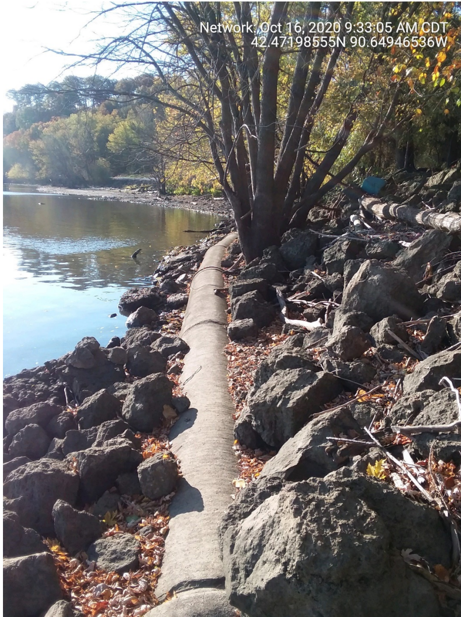
Photograph 6: 10/16/20, Study Area, Exposed Forced Main, Looking South
