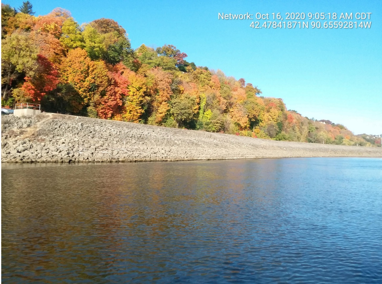
Photograph 1: 10/16/20, Study Area South End, Looking Northwest
