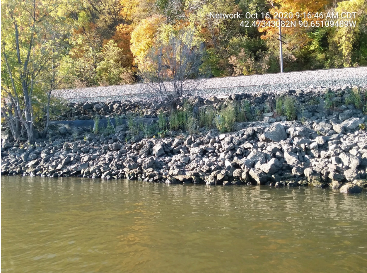
Photograph 3: 10/16/20, Study Area, Mid-Section, Looking Southwest
