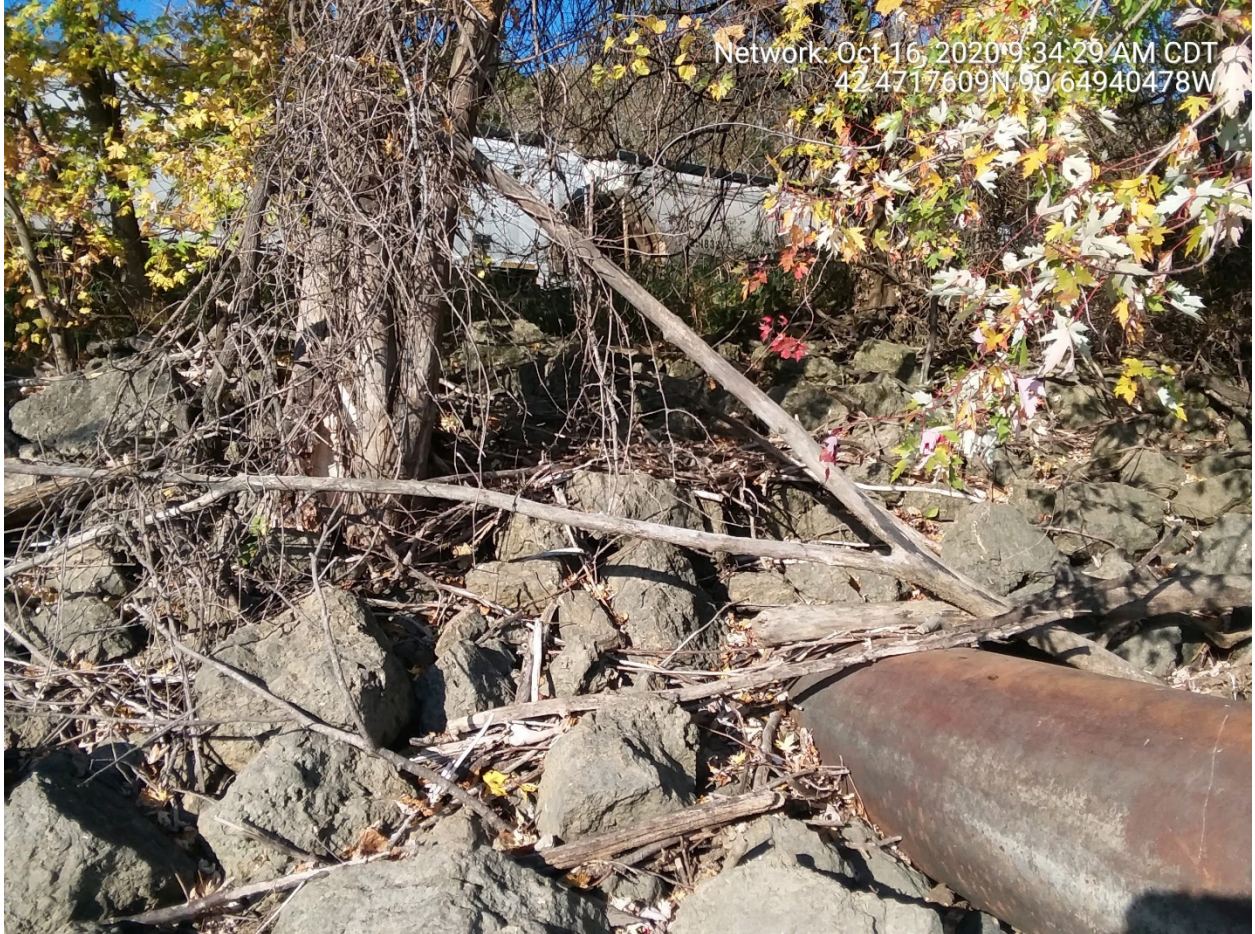
Photograph 8: 10/16/20, Study Area, Close Up of Riprap
