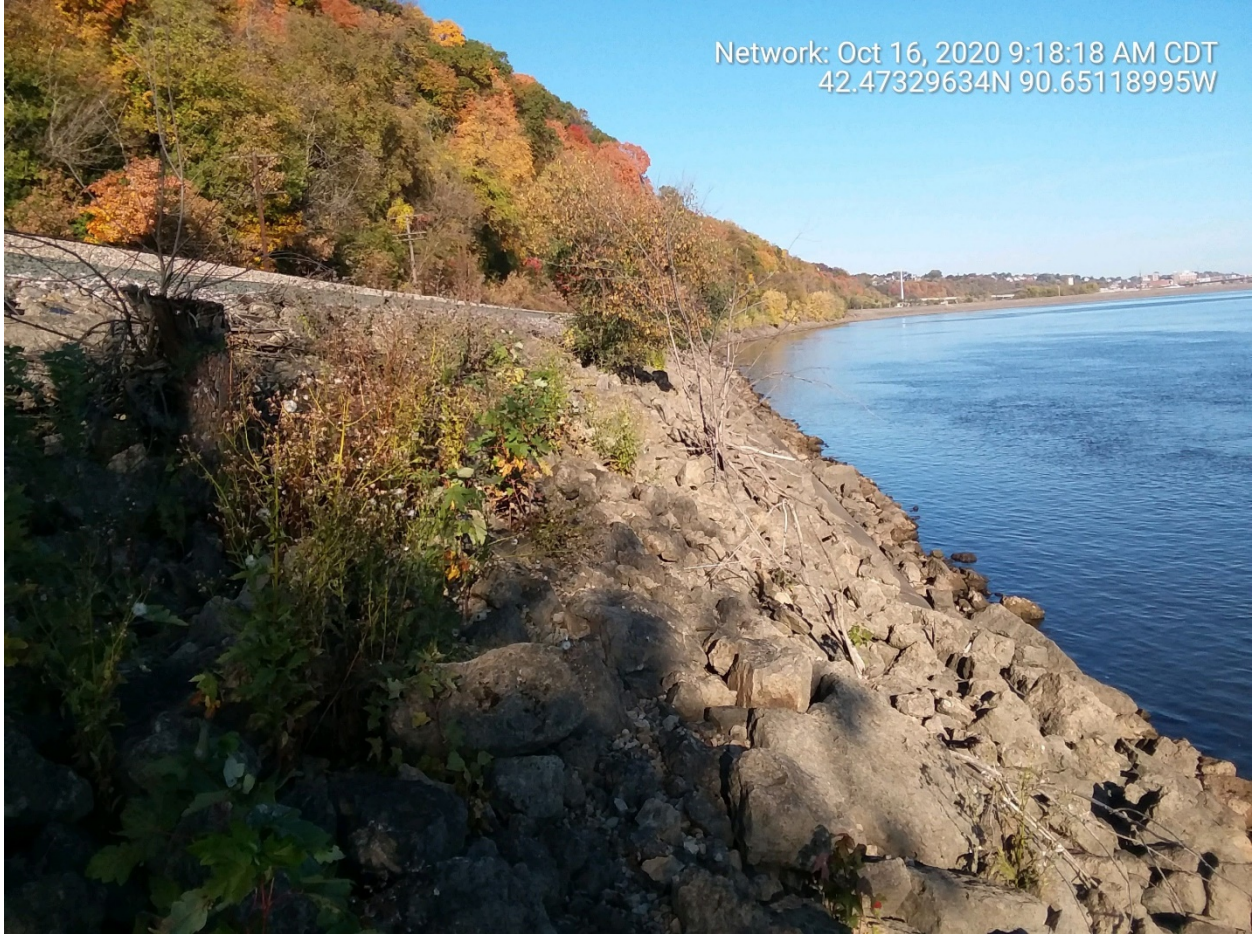
Photograph 4: 10/16/20, Study Area, Southern End, Looking North-Northwest
